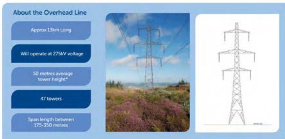
Plate 2.1: Overhead Line Details
